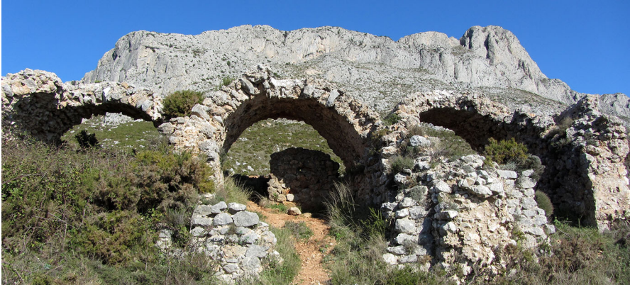
Fig. 7 Surviving vaults of the ancient quarters of the soldiers. Photo by Silvia Bertacchi
